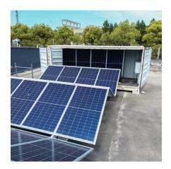
Now, to determine the appropriate solar panel fuse size, we have to first find the maximum short circuit current (Isc) of the panels. You can usually get this value on the panel"s sticker at the ...
