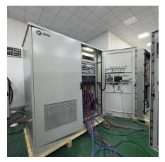
A battery energy storage system (BESS) or battery storage power station is a type of energy storage technology that uses a group of batteries to store electrical energy.
