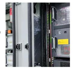
storage system solution. It provides a cabinetlevel battery management system and supports a maximum of 15 cabinets ...
